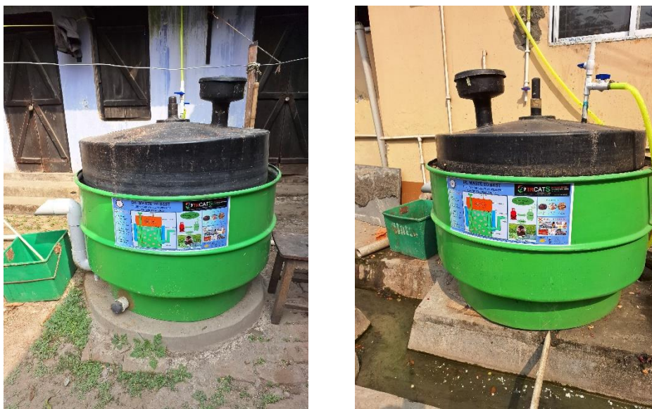
Fig. 11 Biogas systems installed in the College Campus
